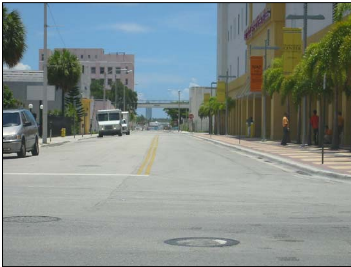
Miami, Florida - NE 9 th Street, at Miami Avenue looking east
