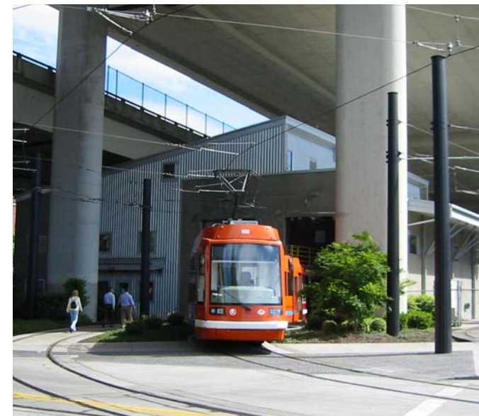
Portland, Oregon—Maintenance and Operations Facility
